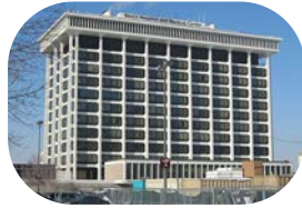
Insight Hospital & Medical Center (Chicago, IL)
